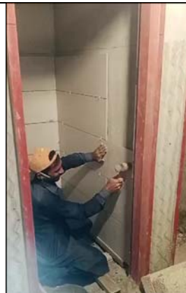
Washroom Tiles Fixing
