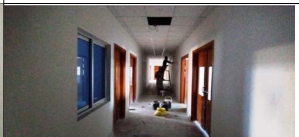
Maintenance of Corridor, Classrooms and offices
