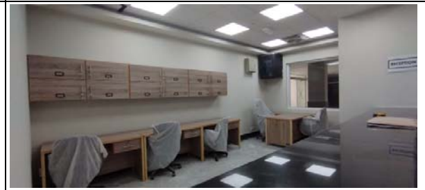
Installation of New Furniture
