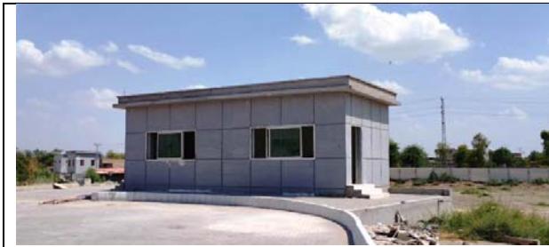
Maintenance of Fire Safety Department
