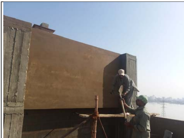
Water tank maintenance at ZU Clifton Site
