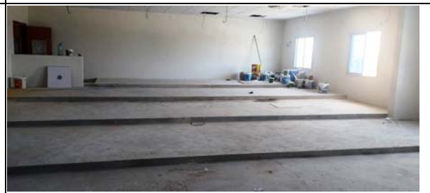
Renovation of Lecture Halls
