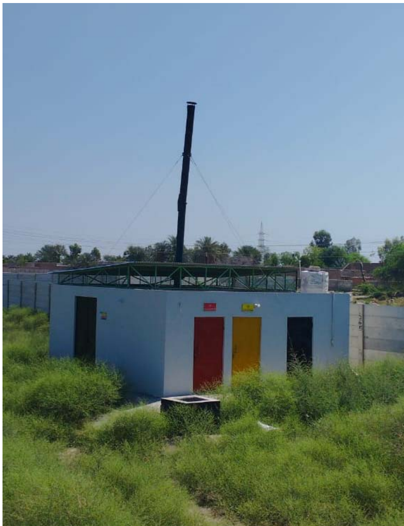
Incineration Room for handling, disposing and recycle of waste
