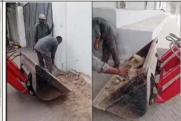
Internal Parking Area Maintenance
